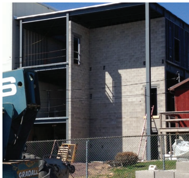
The new home for Citterio USA's slicing department takes shape in Freeland, PA.
